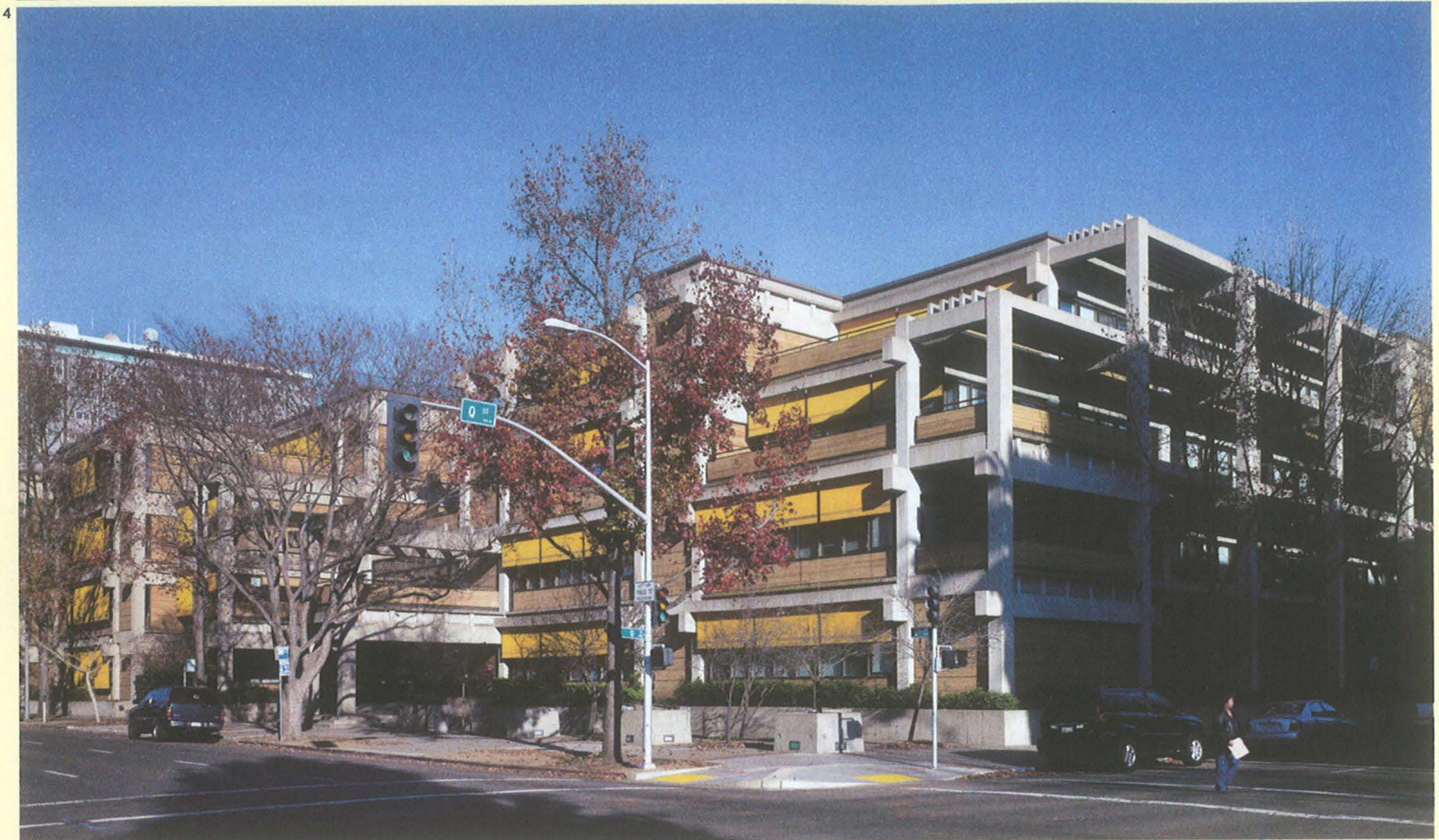
4. Bateson Building south-west view with the yellow vertical canvas blinds. The south elevation illustrates the horizontal concrete baffles which are spaced apart to provide airflow but cut the summer sun angles
